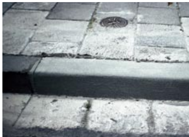
Renovation of kerbstones with SILIKAL® R 17 mortar
