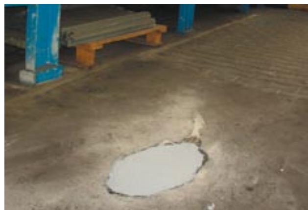
Renovation of flooring in a rolling mill
